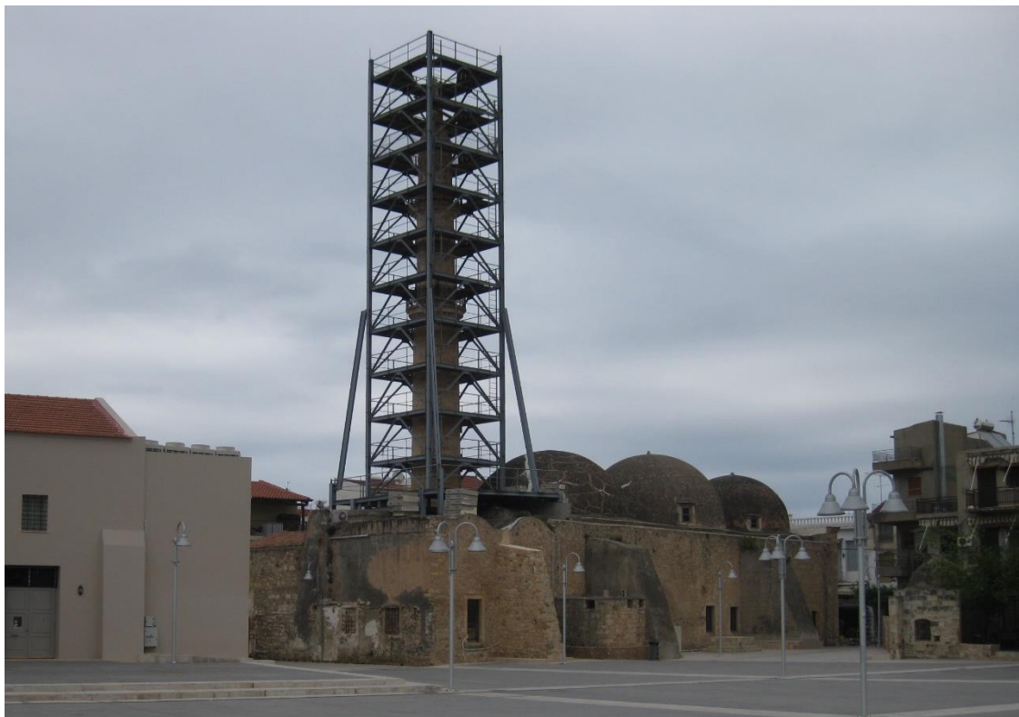
IMG_0373, 24 April 2009 S. Maria degli Agostani, showing the minaret during restoration (now completed) as well as the domes that were added in the Ottoman period.
