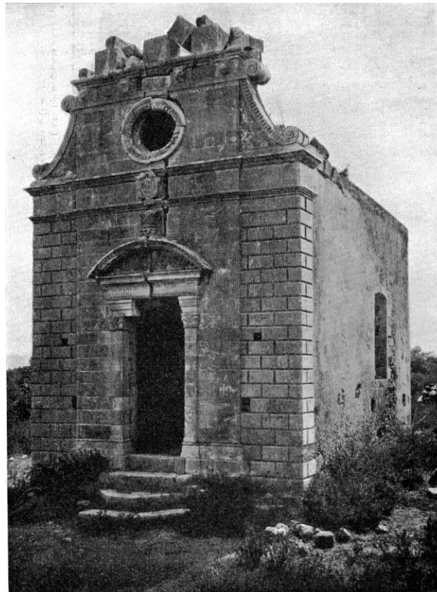
Gerola's photo (II 292) showing the church before restoration (and the addition of the concrete belfry).
