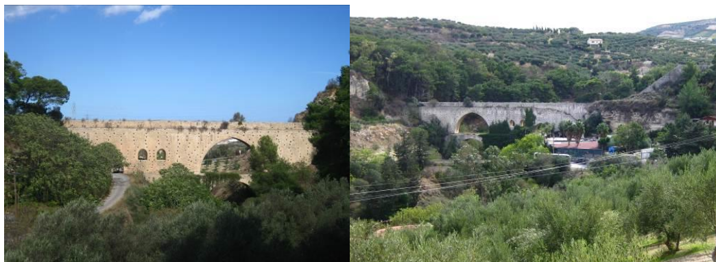
(left) IMG_2731 The aqueduct (Dawkins' no. 1) that was built (or restored) under Egyptian rule in 1839. 29
