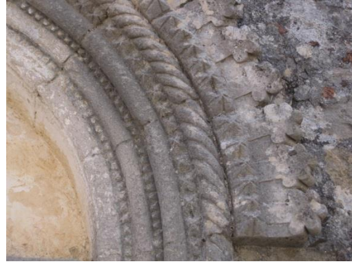
IMG_8078 Moulding on W door
