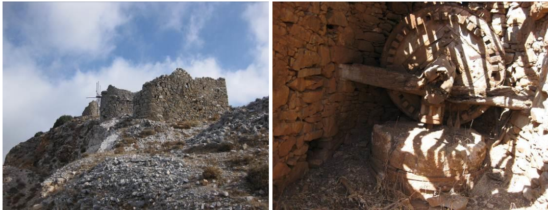
(left) IMG_5199 Ruined windmills at Seli Ambelou (northern entrance to Lasithi) (right) IMG_5095 Remains of toothed wheel and “lantern” in ruined windmill as described by Dawkins (near Kardamoutsas Monastery: see ch. 27)
