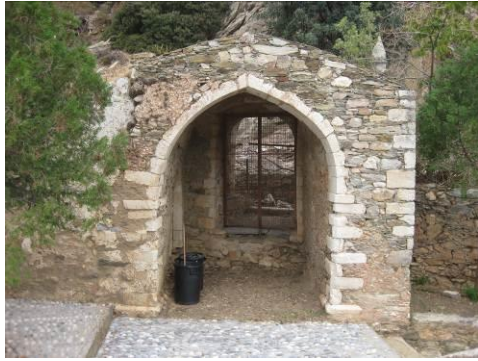
IMG_2776 The inside of the former gateway showing one of the miniature pyramidal decorations
