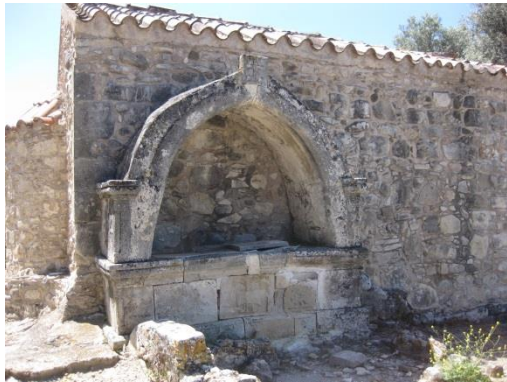
IMG_8137 North wall
