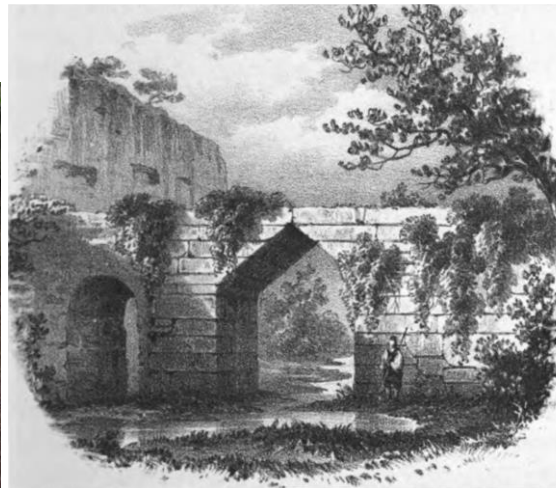
Upper bridge (Spratt II 95)
